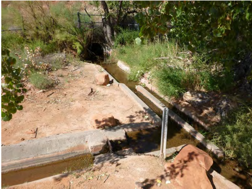
Concrete-lined ditch east of I-15
